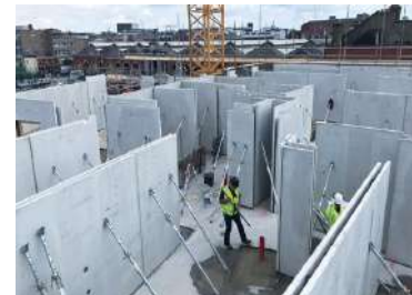
Fig 102 : Twin wall Technology
