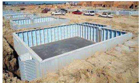
Fig 100: Precast Concrete Foundation
