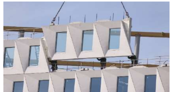
Fig 101 : precast flat panel system
