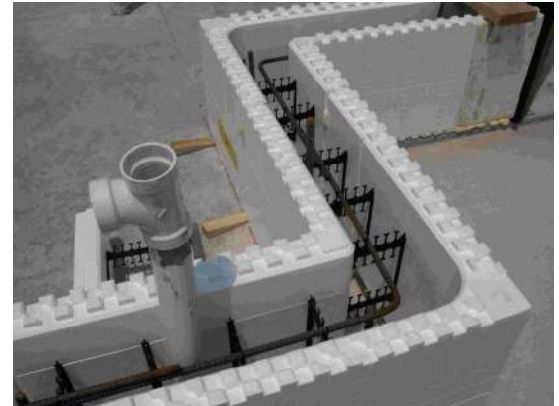
Fig 99 : Insulating concrete formwork
